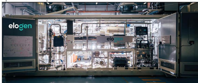
Figure 2 : 1.2 MW containerized PEM water electrolyzer (courtesy: Elogen Co.).
